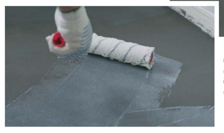
It has high elasiticity qualities, adheres itself strongly to cement or clay surfaces and avoids fluoresence (saltpeter) by protetcting the superficial layer and increasing the sealers life.
